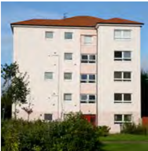
This block of Local Authority-owned flats benefitted from a flat to pitch conversion using Metrotile roofing.
