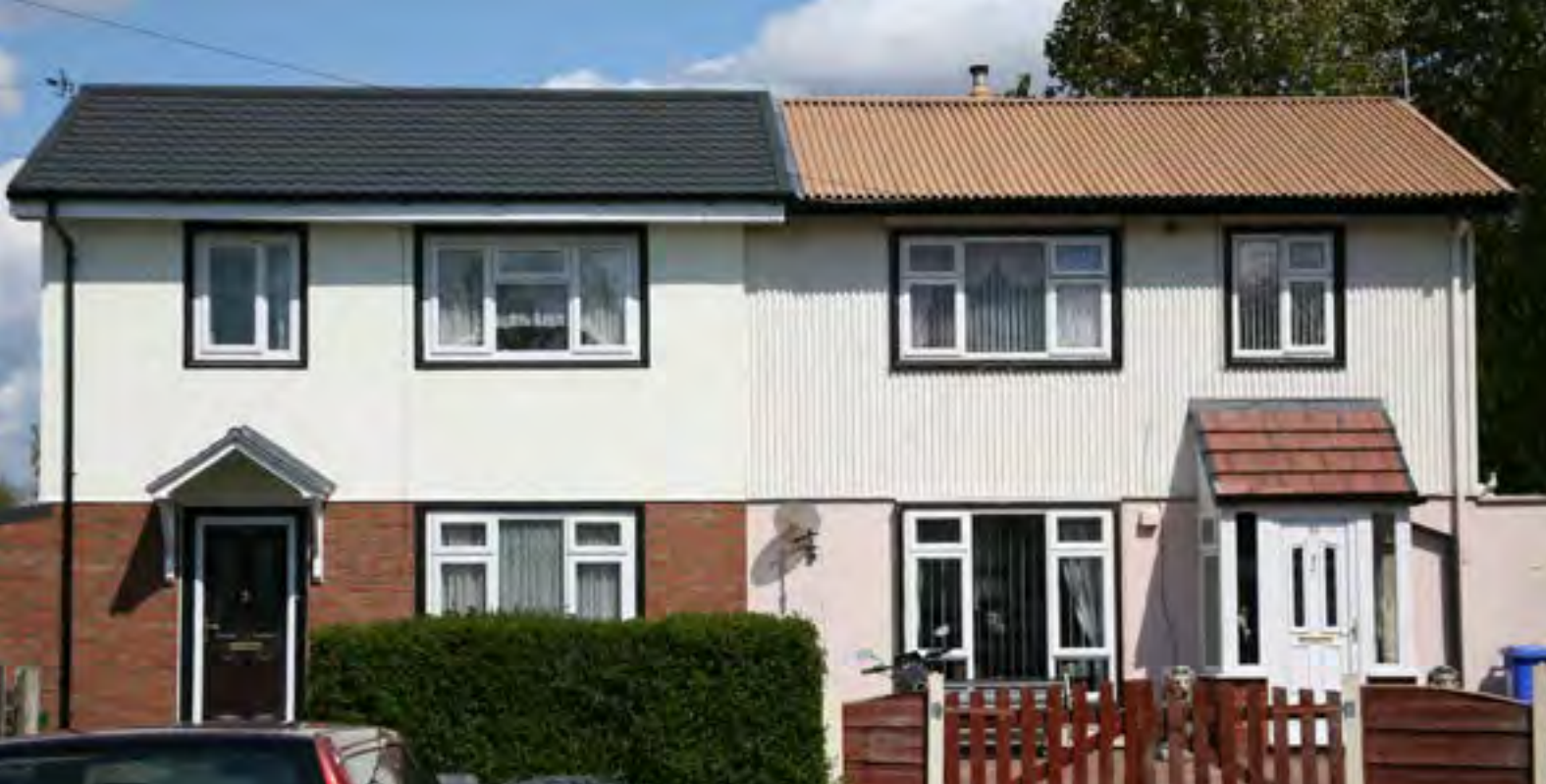
Two BISF homes showing a newly refurbished Metrotile roof against the old.
